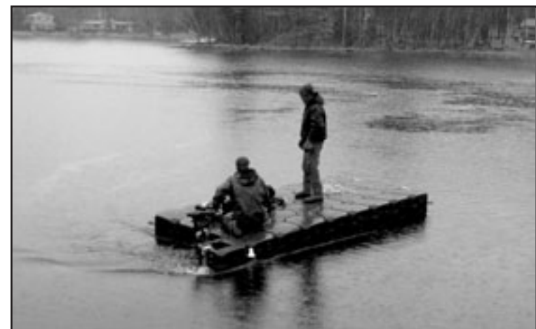
Working on the valve.
